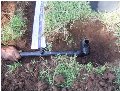
Dig hole for flush valve
