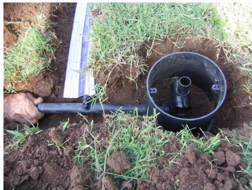
Protect valve with valve box
